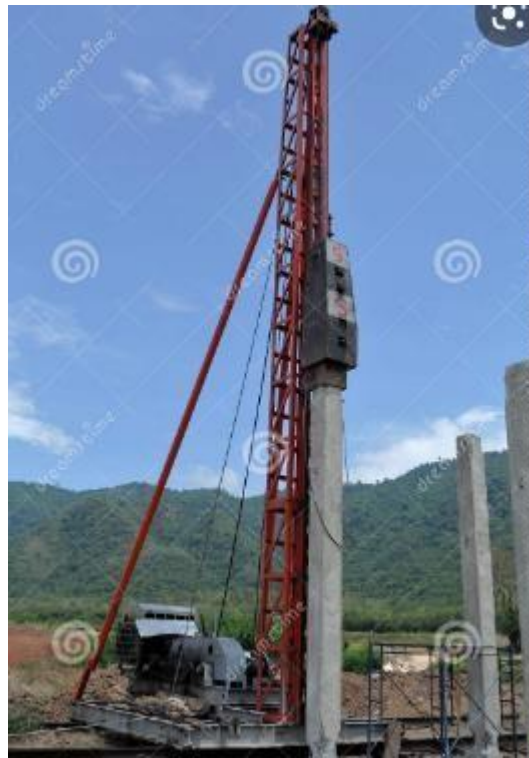
Figure-1: Pile driving using hammer
